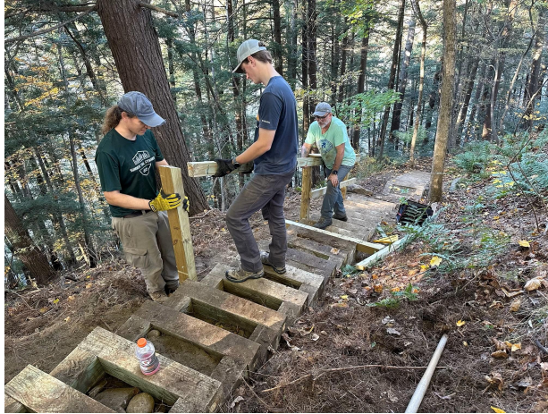
Example of wooden steps.
